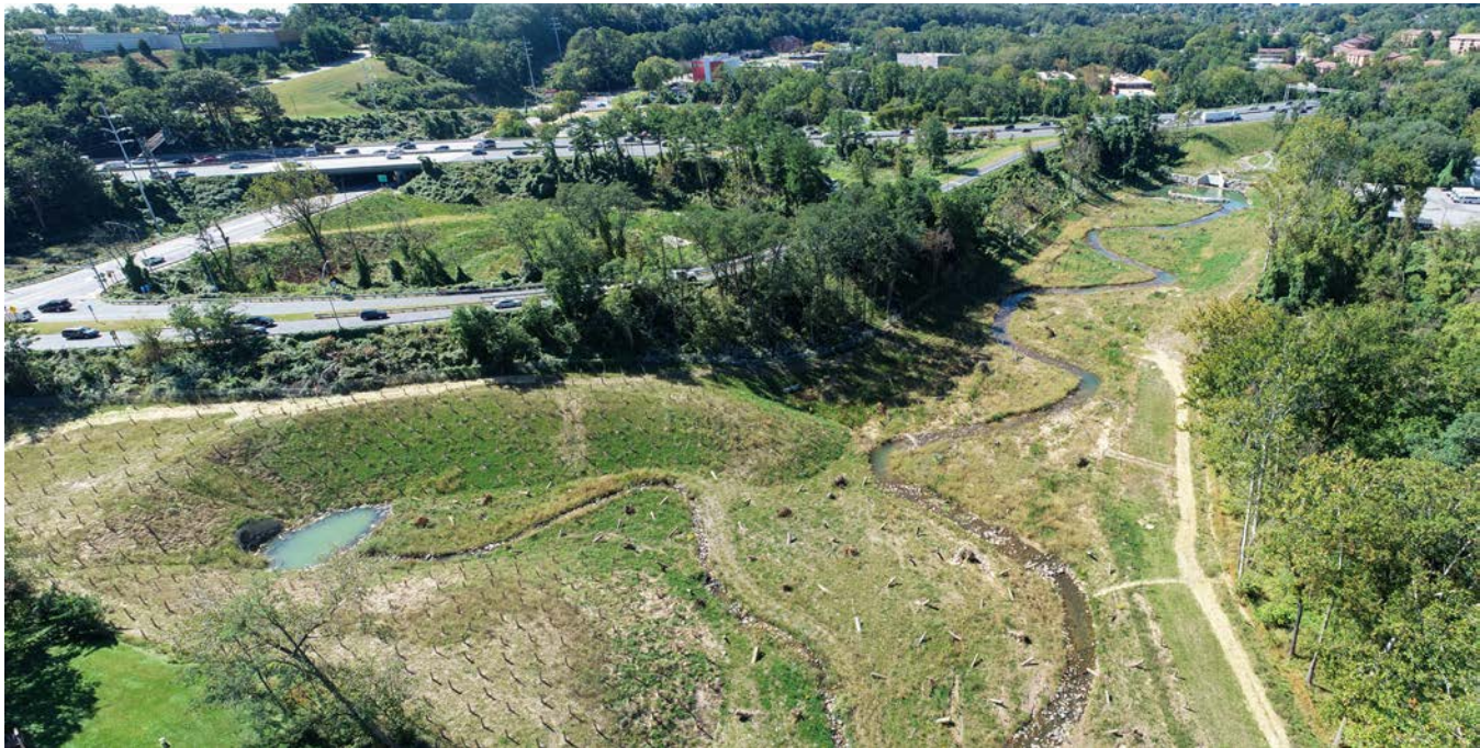
Minebank Run Stream Restoration and Water Quality Improvement Project, located along I-695 at Cromwell Bridge Road north of Baltimore, was completed in 2021 for Maryland State Highway Administration, and included stream and floodplain restoration, outfall stabilization, wetland creation, reforestation, and stormwater management.
